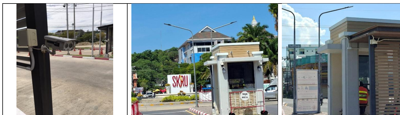
CCTV in entrance (Songkhla Rajabhat University)
