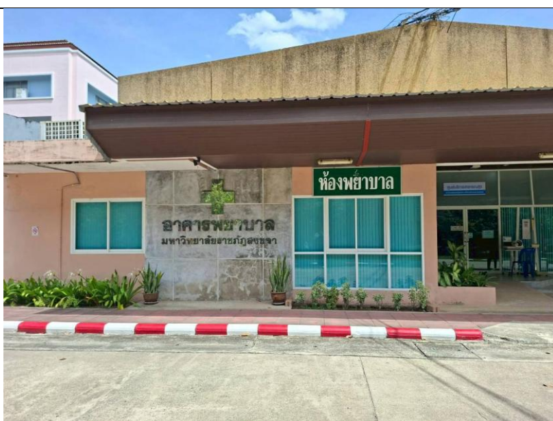
The Infirmary Building, Songkhla Rajabhat University (Songkhla Campus)
