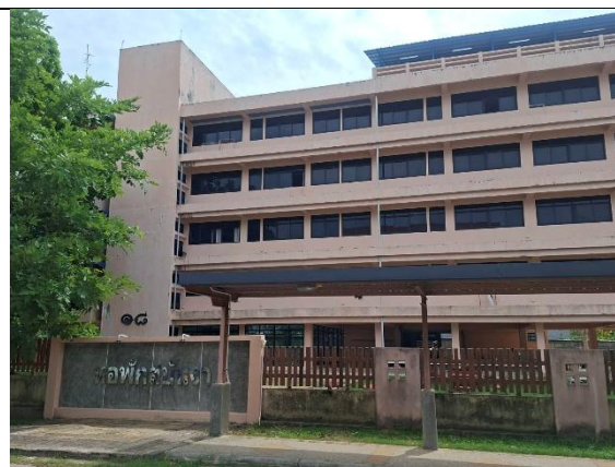
Building 18: Sabanga Student Dormitory Area: 2525.25 m^2
