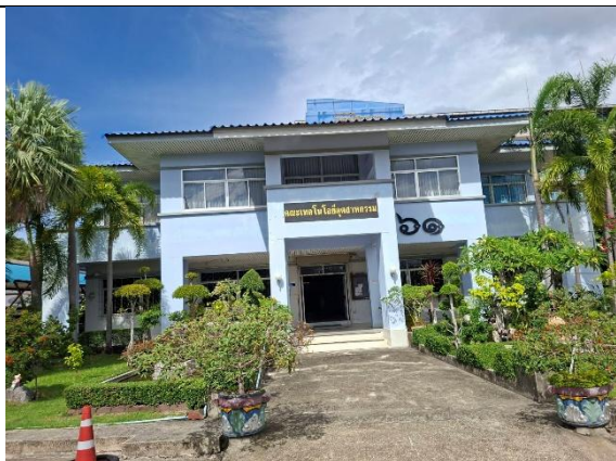
Building 61: Academic Services and Laboratory, Faculty of Industrial Technology Area: 1294.24 m^2
