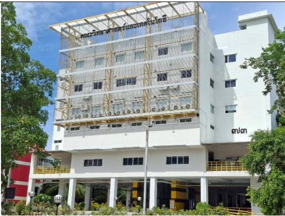
Building 73: Faculty of Science and Technology (Classroom & Laboratory) Area: 27876.00 m^2
