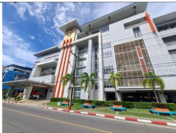
Building 66: Faculty of Management Sciences Area: 29856.00 m^2
