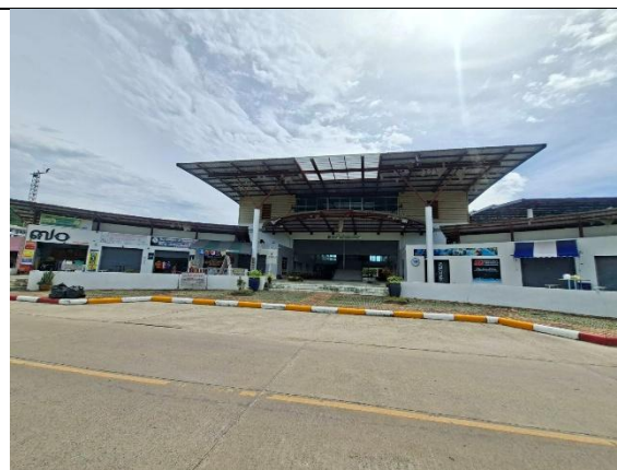
Building 70: Swimming Pool Complex
