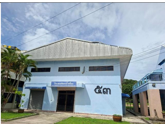
Building 53: Water Production Plant
