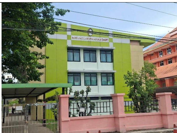
Building 17: SKRU Demonstration School Office Area: 2676.00 m^2
