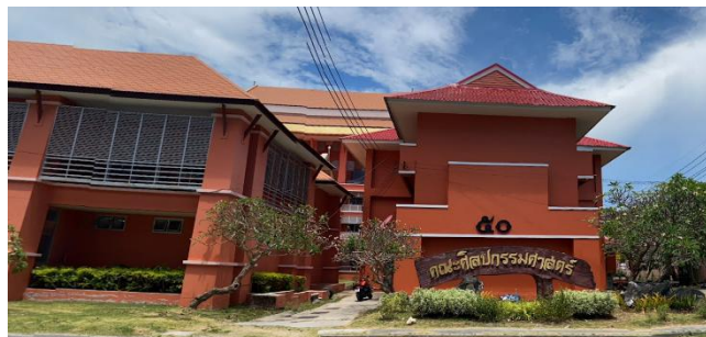
Building 50: Faculty of Fine and Applied Arts
