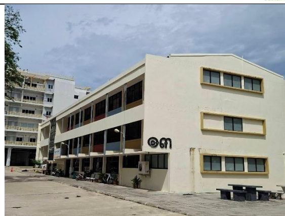
Building 13: Rukkhawan Student Dormitory Area: 1200.00 m^2
