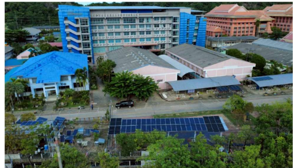
Faculty of Industrial Technology Building No.74 : Solar cell 20 kW
