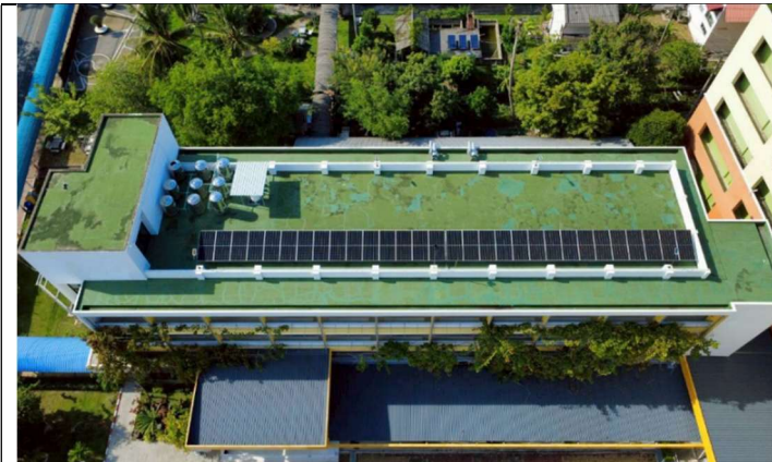
Faculty of Science and Technology Building No.10 : Solar cell 16.5 kW
