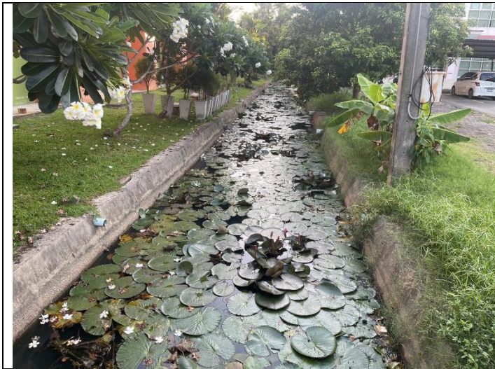
Treated water pond with aquatic plants functioning as an ecological water polishing and retention system within Songkhla Rajabhat University.
