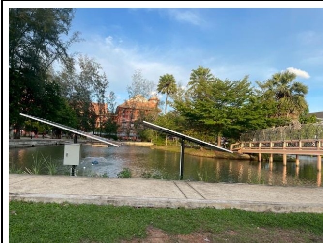
Solar-powered aeration systems in open drainage channels, campus canals, and retention ponds at no fewer than 30 points.
