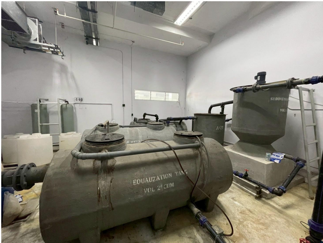
Wastewater treatment system installed in the Faculty of Science and Technology building, which contains teaching and research laboratories.
