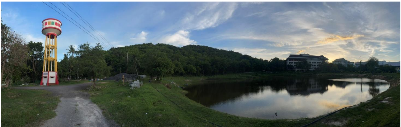
Retention ponds and stormwater storage areas at the Main Campus.
