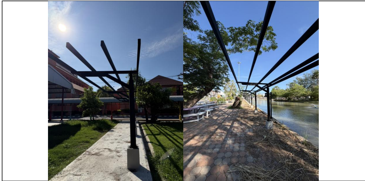
Figure: Songkhla Rajabhat University is currently constructing an additional 198-meter covered walkway to connect the motorcycle parking area at Gate 1 with the inner campus pedestrian network. This project will improve pedestrian safety, provide weather-protected walking access, and encourage students and staff to walk instead of using motorcycles or private vehicles for short-distance travel. The construction of this covered walkway demonstrates the university's continuous effort to enhance pedestrian-friendly infrastructure.
