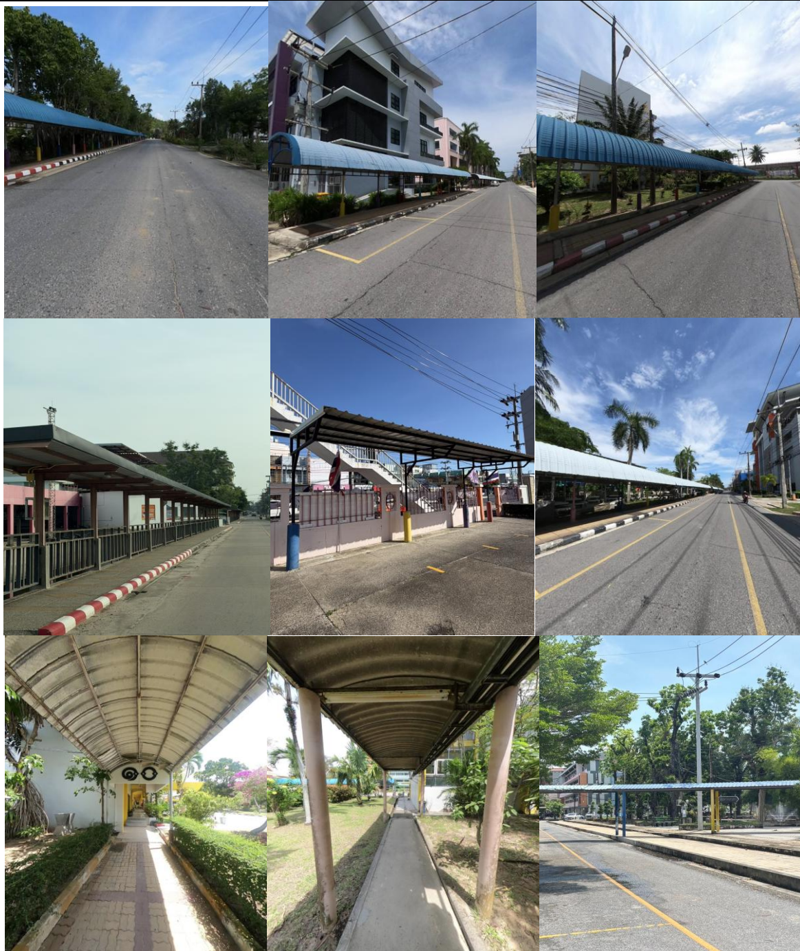
Figure: Songkhla Rajabhat University has continuously expanded covered walkways on campus to support safe, convenient, and weather-protected pedestrian movement. These covered pedestrian paths connect important areas of the university and encourage students, staff, and visitors to walk instead of using private vehicles for short-distance travel. This initiative helps reduce car use, lower traffic congestion, promote healthy mobility.
